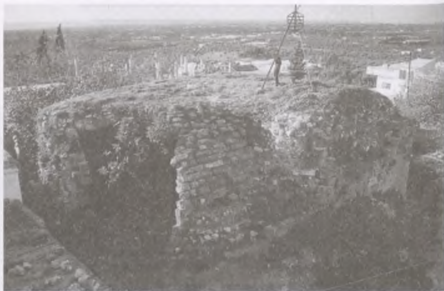
1. Burğ Mi'ār Šākir – ground floor of the tower from the southeast
