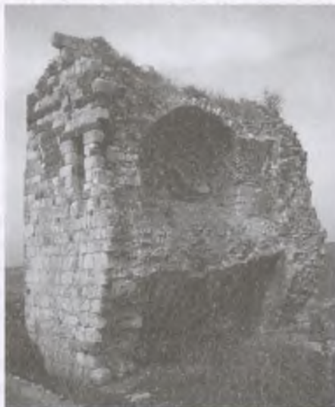
3. Qal'at Umm Hūš - the tower from the southeast
